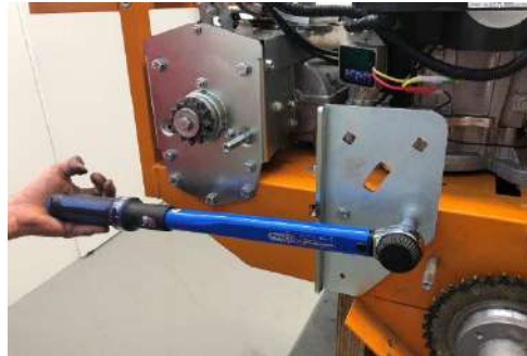
Mount new chain tensioning plate.
